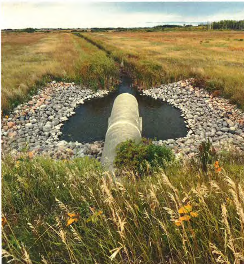
Pipe outlet – riprap plunge pool
