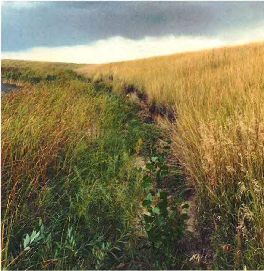
Erosion on pool side of north embankment.
