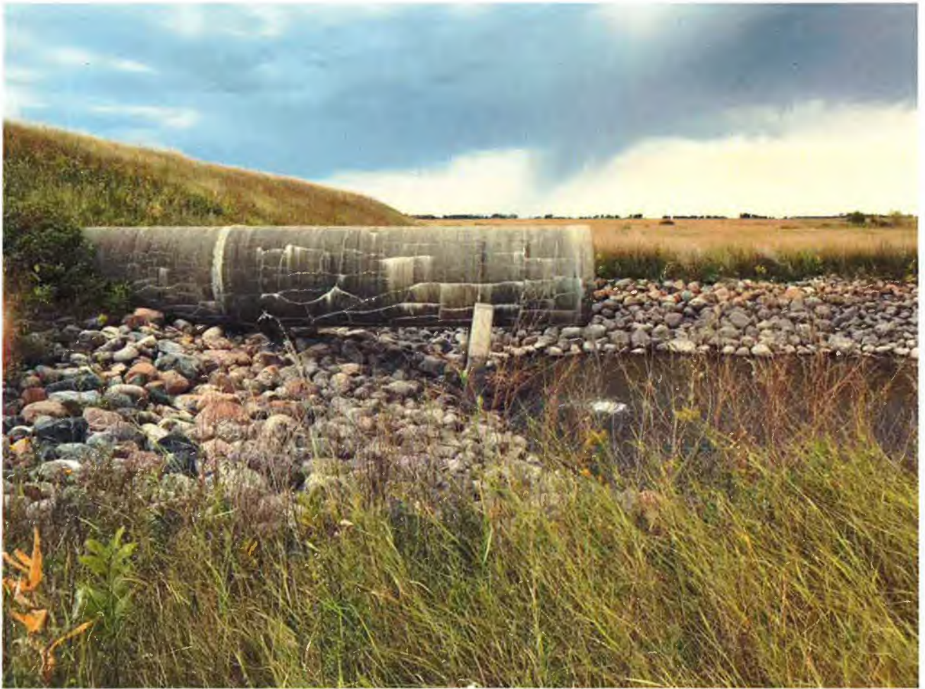
Pipe prop tilted. Appears no worse than when first identified
